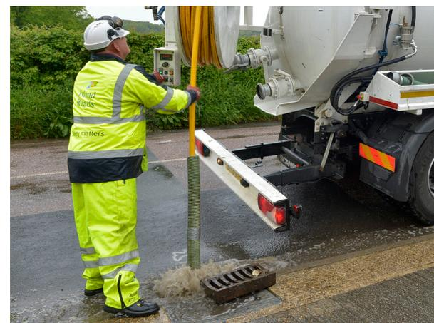
We also have a specialist drainage team working on a scheduled programme to cleanse and repair all gullies and drains across the Island ahead of our surfacing works. This work will repair systems that have suffered from years of poor maintenance due to the lack of funding.
